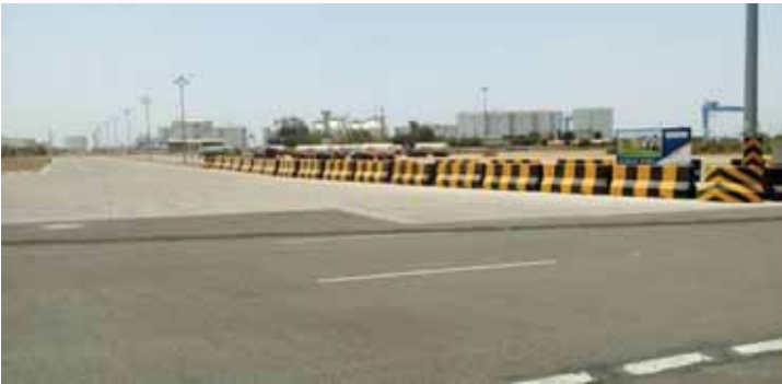
Port Pipavav, Gujarat
