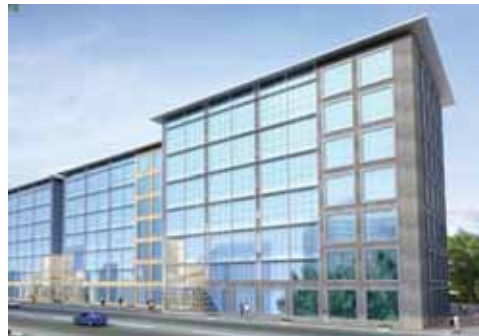
Kohinoor Commercial Complex, Mumbai
