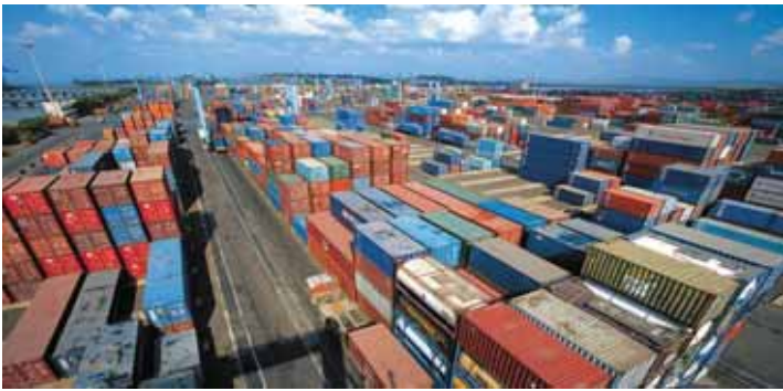
Nhava Sheva International Container Terminal (NSCIT)
